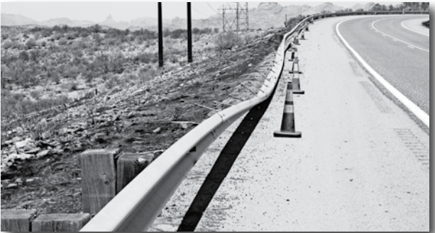
The guard rail posts were burned in several places on Hwy. 177 between Kearny and Superior. James Carnes | Copper Area News
